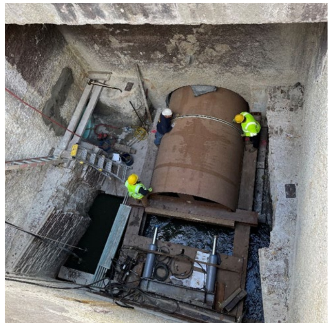
Rehabilitation of the NBMI – Phase I – Sliplining in Andrew Square
