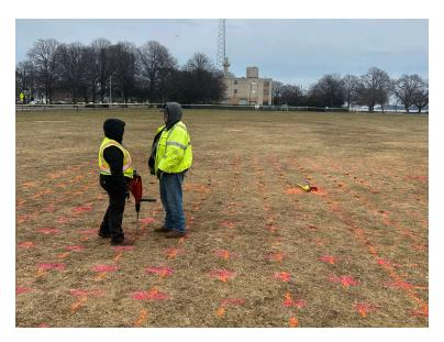
After crews could not locate buried manhole in Moakley Park by metal detector, a grid was painted to guide drilling exploration.
