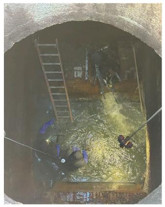
Initial cleaning of the existing NBMI pipe through Special Manhole B in Moakley Park.
