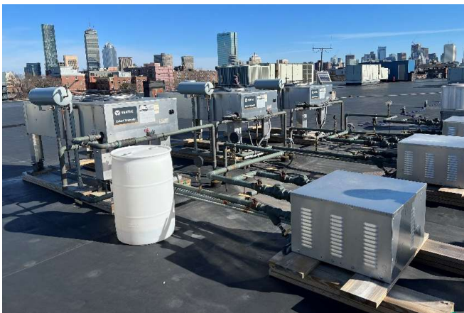
Removal and Replacement of Roof Top Units
