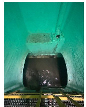
Special Manhole B AFTER
