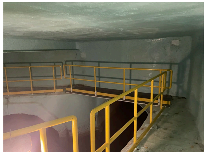
Rehabilitated Special Manhole A
