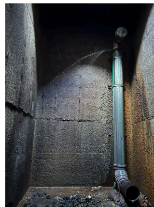
Special Manhole B BEFORE
