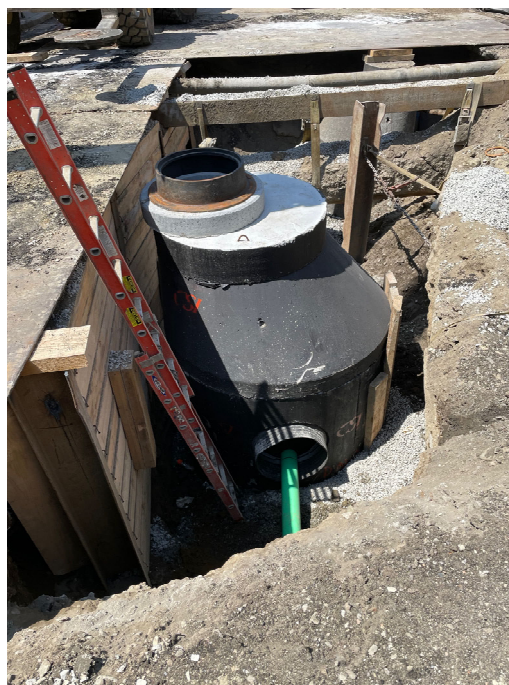
Manhole installation in West Seventh Street
