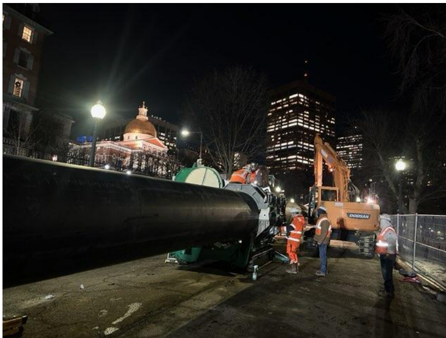
19-308-004 Water Main Replacement in Beacon Hill
