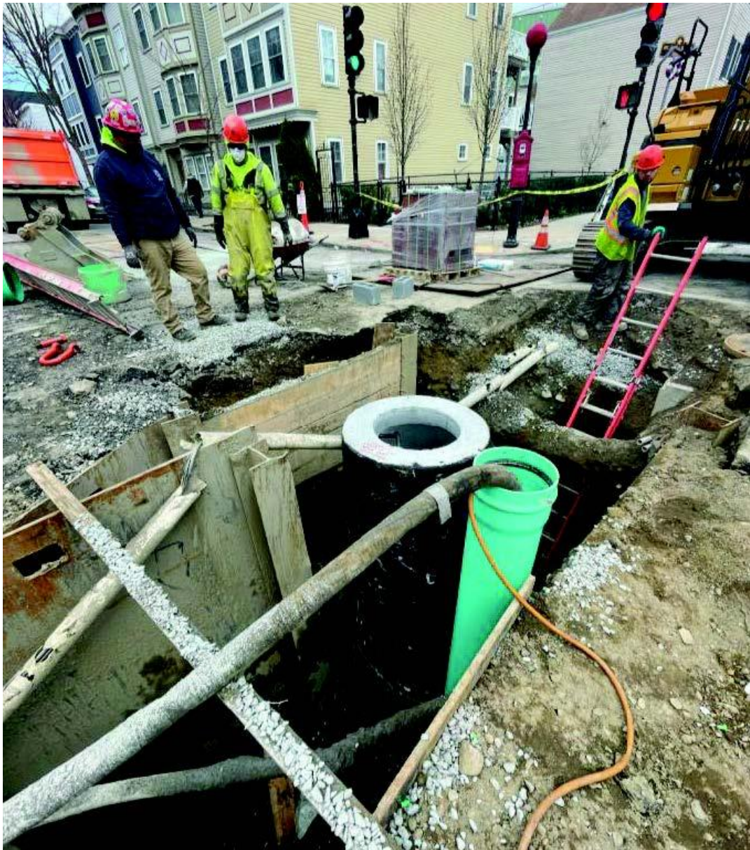
22-309-012 Sewer Manhole Installation on West Seventh St. at D St.
