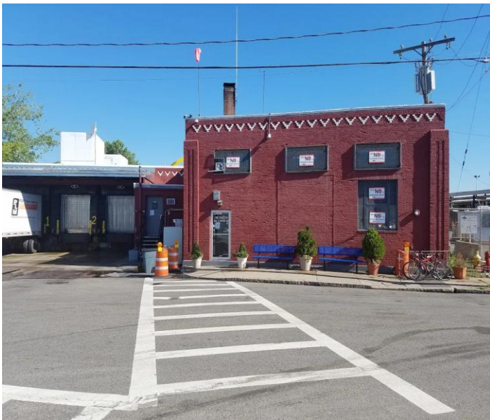
Channel Fish Loading Docks at East Eagle Street
