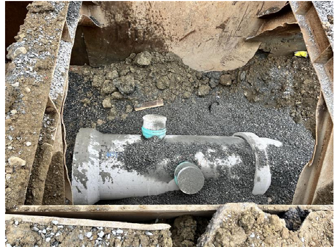
Drainpipe with catch basin connections in West Fifth Street
