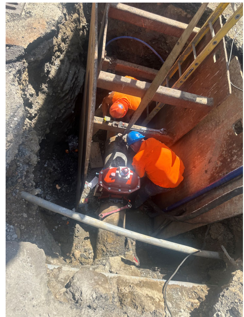
Gate valve installation in West Fifth Street
