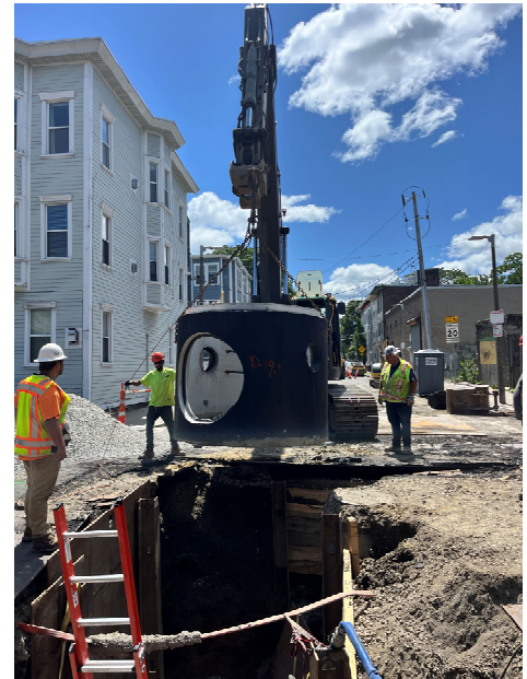
Drain manhole installation in West Fifth Street
