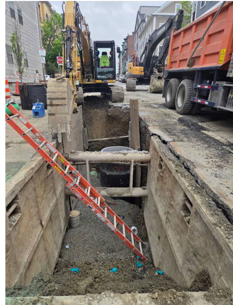
Drain manhole installation in E Street
