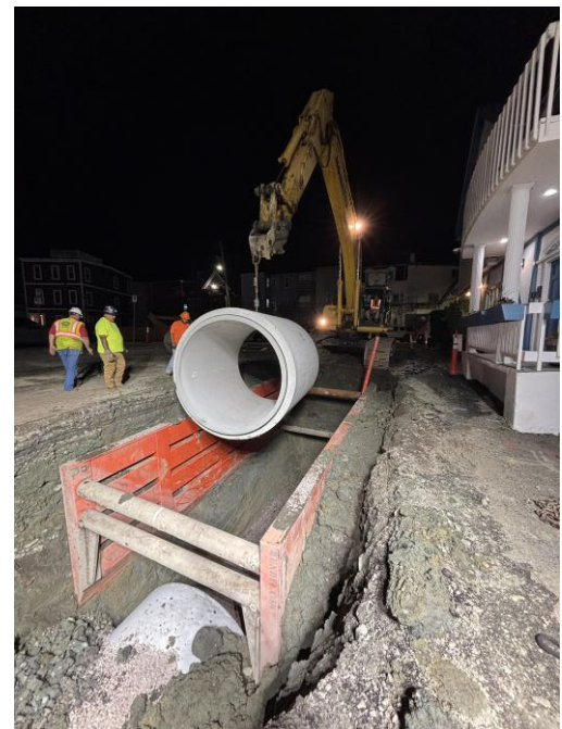
Drain installation in Eagle Square
