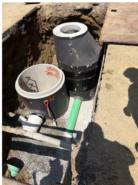
Sewer and drain manhole installation in E Street
