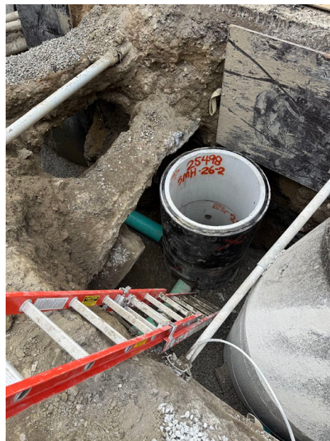
Drain manhole installation in E Street
